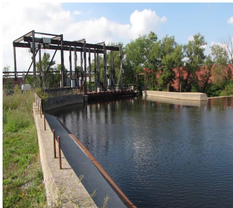
1.9-MW Tannery Island hydro facility Source: Ampersand Hydro
